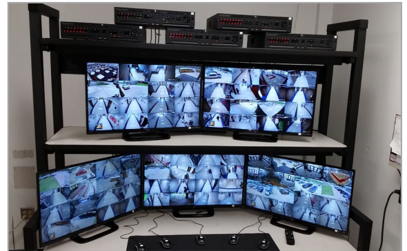
The new security cameras are installed and running at Sam Houston High School, the first AISD high school to receive the new cameras.
