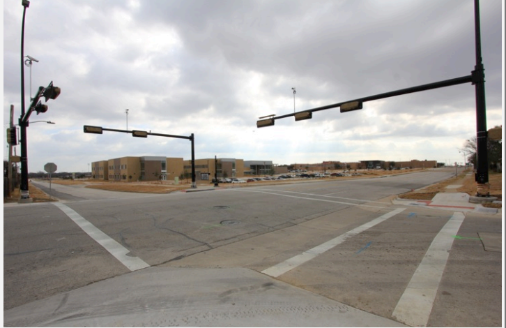
McNutt traffic signal
