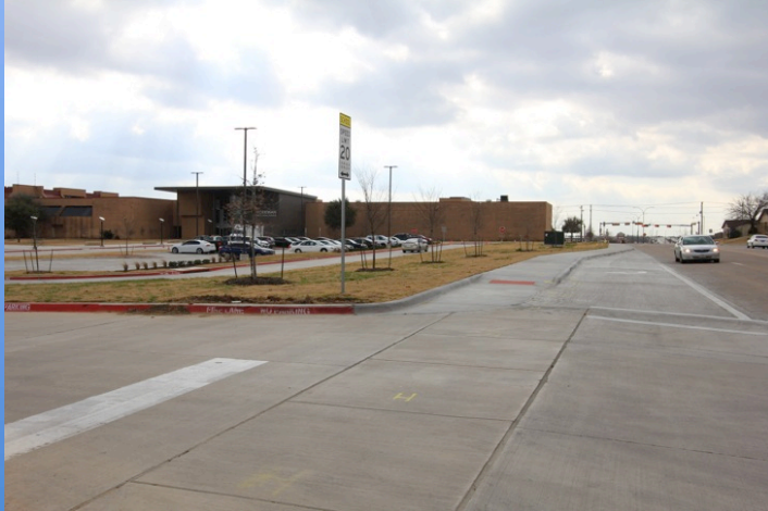
Workman decel lane
