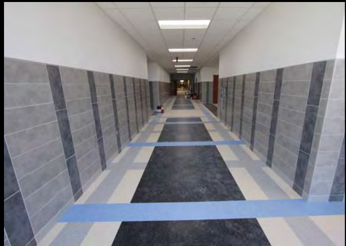
Seguin High School – renovated dance room, addition hallway
