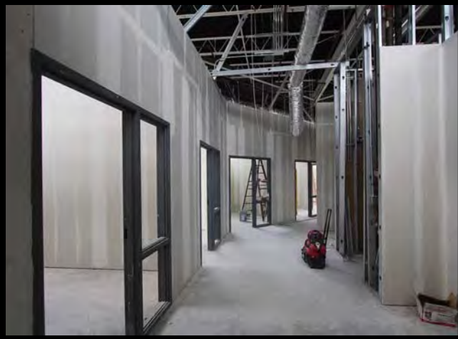
Goodman – admin renovations
