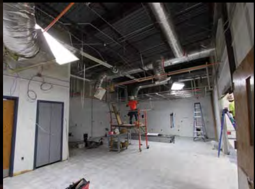
Sam Houston High School - auditorium, band renovations
