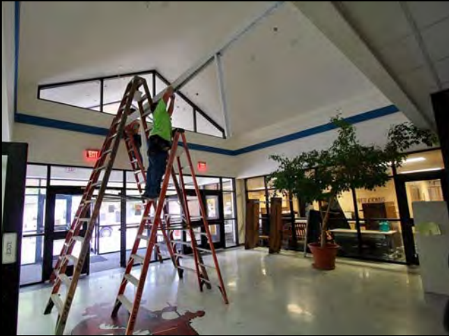
Dunn – entrance renovations and security vestibule
