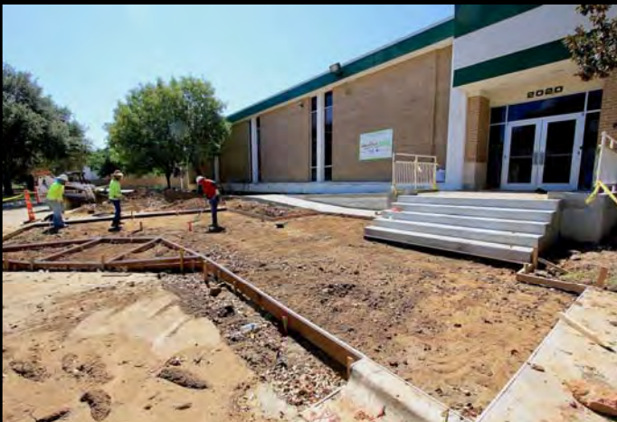
Hill – sidewalks and ramp
