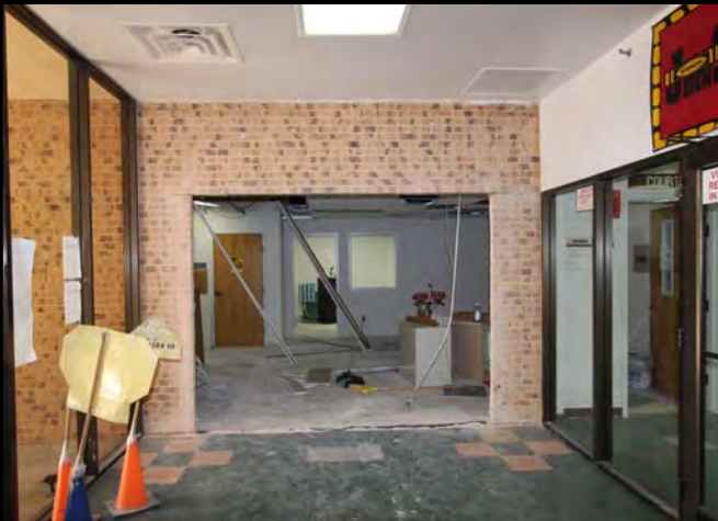
Johns – reception and security vestibule renovations
