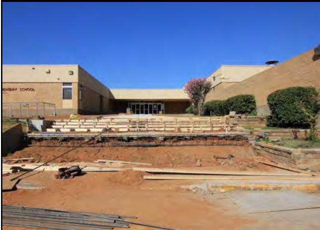
Sherrod – sidewalks, stairs and parking lot
