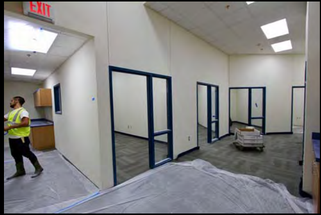
Goodman – admin renovations
