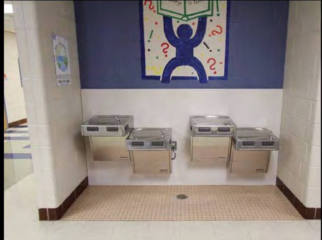
Roark – new water fountains
