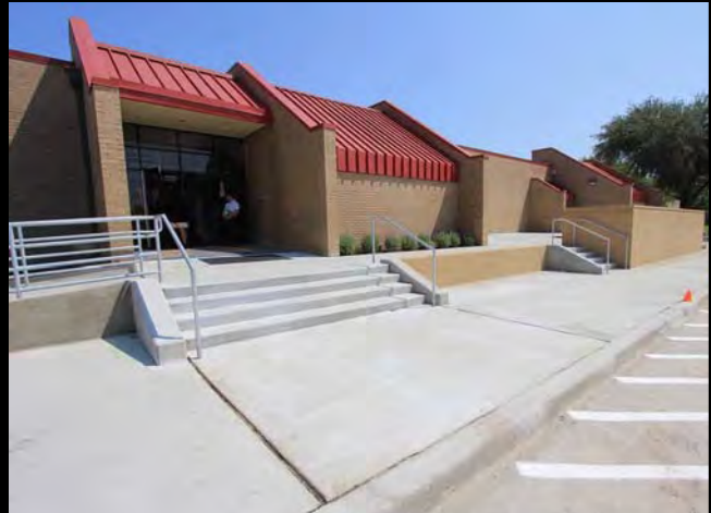
Atherton – front concrete
