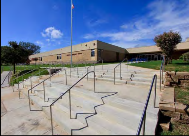
Sherrod – sidewalks, stairs and parking lot
