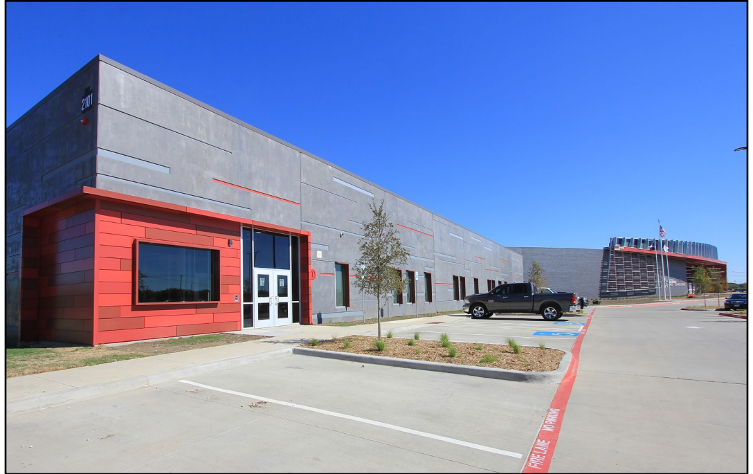
The new data center has been running as planned for the last year.
